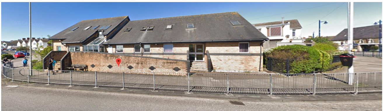
Hillsboro Place Car Park
